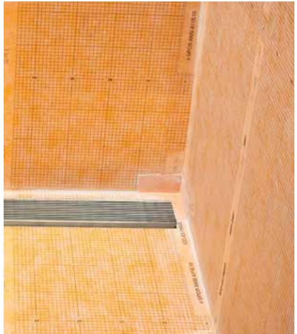
½" Flange with Schluter®-KERDI available for Next Day Custom Exactly Wall to Wall, Flush Against the Wall®
