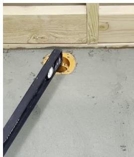
**Spread a primary mortar bed across the intended shower area. Pitch this bed in all directions towards the drain body.**
