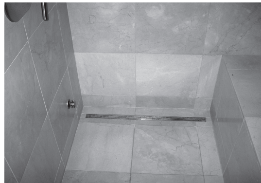
Fig 3 S-AG 38 installed NOT wall-to-wall. If the drain does not finish wall-to-wall the remaining area must have flooring material on either side and have pitch back to the drain.
