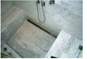
Fig 1: S-AS 65 finished wall-to-wall with build out.
