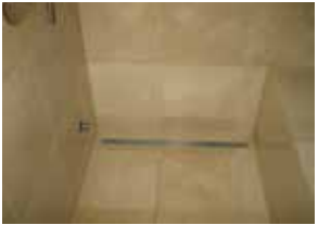
Fig 2: S-AG 38 installed NOT wall-to-wall. If the drain does not finish wall-to-wall the remaining area must have flooring material on either side and pitch back to the drain.
