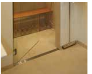
Fig 5: Threshold Installation FFED 65 where the entire bathroom is waterproofed. The dry side is slightly pitched towards the linear drain.
