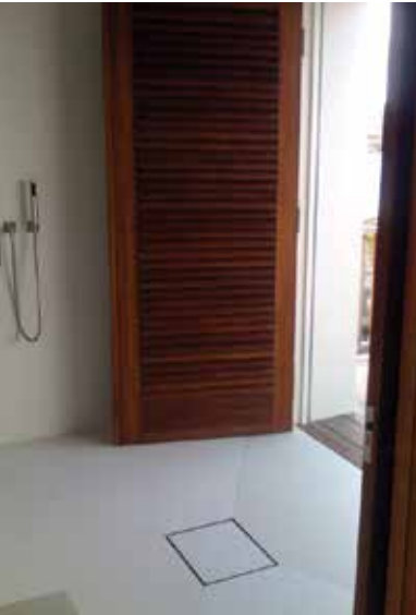
Size 5"x5" 16 gauge, 304 Stainless Steel ABS/SS Body 2" Throat Installation Types: Center Drain (TD) Center Drain (TDB)
