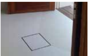
Fig 6: Tile Drain Series: Center Pitch Installation
