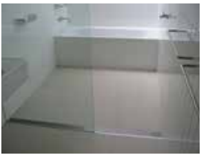
Fig 4: Threshold installation using the S-AS 65 demonstrates an exact wall-to-wall barrier free installation.
