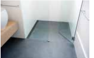
Fig 3: Against the wall installation with the FFAS 65 series.
